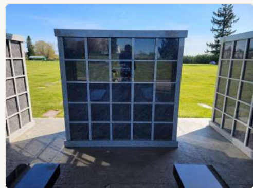
Wall D stands across the head of the courtyard, on its own.
